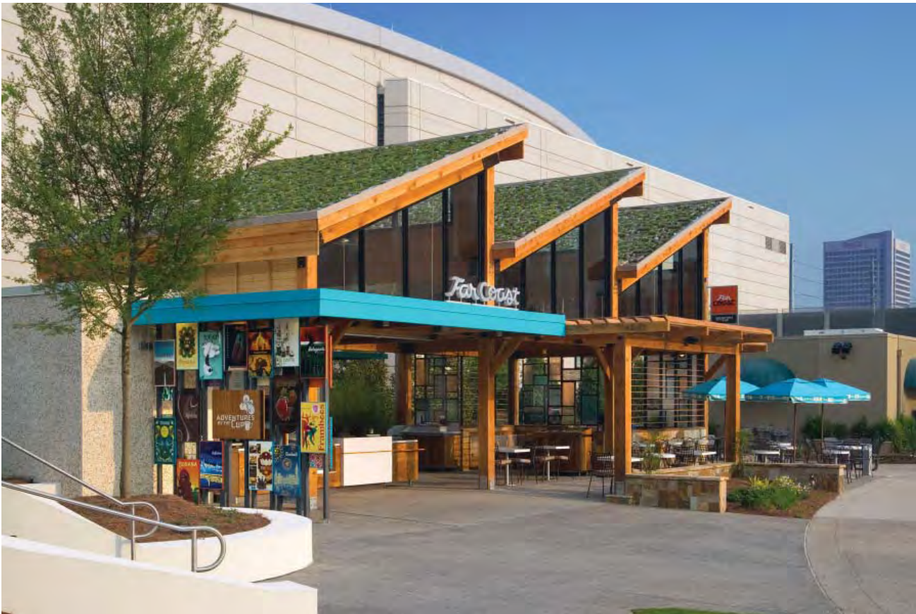
3 southeast exterior pavilion viewing green roof - far coast cafe, atlanta, ga
