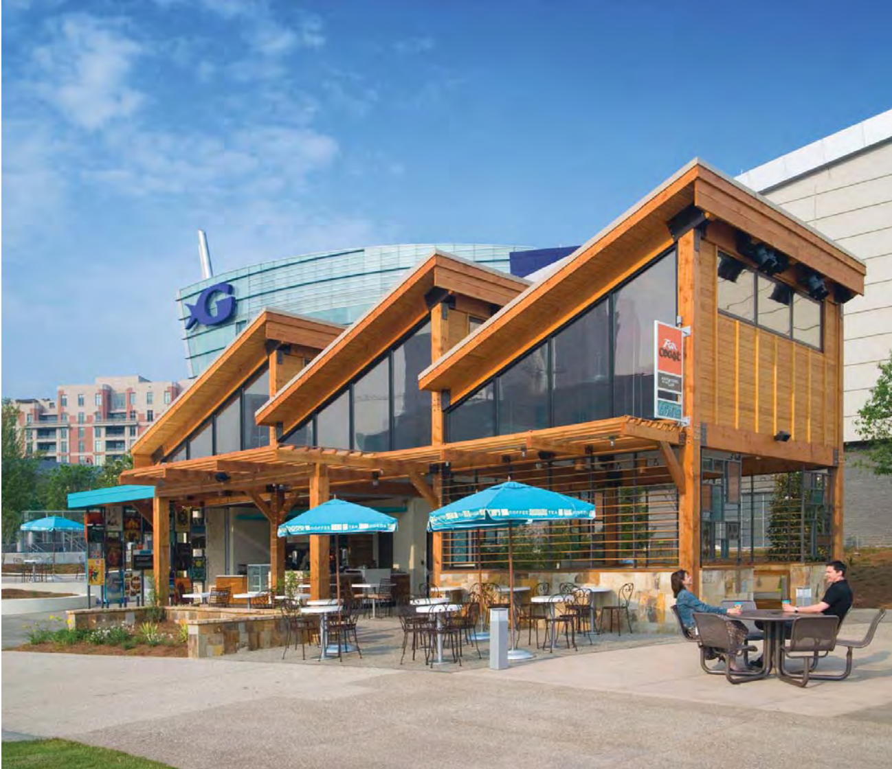
7 northeast exterior in world of coca cola context, georgia aquarium beyond
