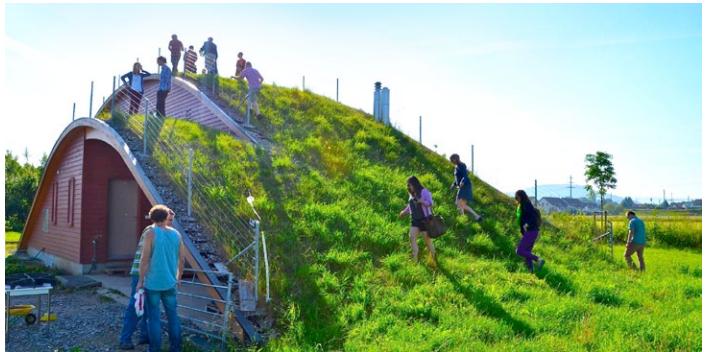
CLOCKWISE FROM UPPER LEFT: Logs and stones provide habitat niches for fauna; planting on Zurich's Sihlcity shopping mall roof; agricultural green roofs, like this one in Mohlin, provide additional area for crops and grazing; a simple overflow system ensures drainage and water transfer between planted roof areas at the Sihlcity shopping mall. Photos: Lisa Lee Benjamin (top left) and Jeff Joslin
