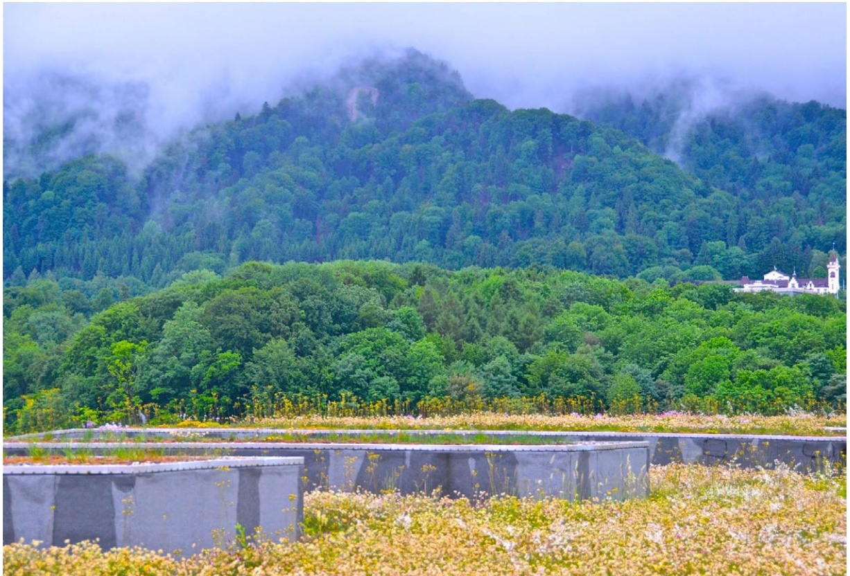
The prolific green roofs of Switzerland’s major cities meld even their most industrial edges with the surrounding landscape. Photo: Jeff Joslin
