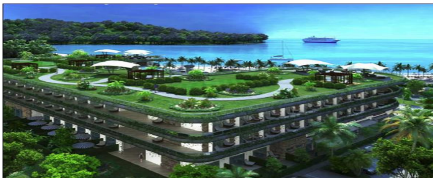
Green Roof | Palazzo Park Hotel & Residences, Manuel Antonio Costa Rica
