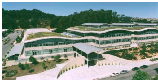
The Gap Headquarters, San Bruno CA, 1997 by McDonough + Partners and American Hydrotech
