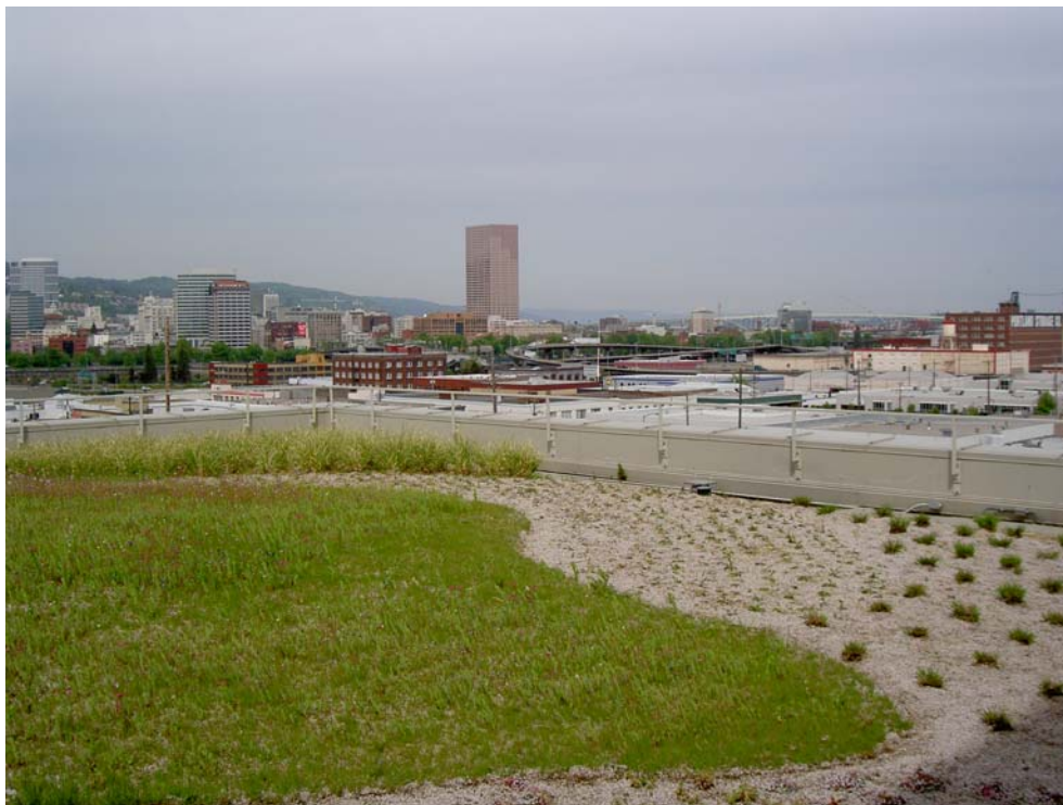
A recently installed ecoroof atop the Multnomah County Building demonstrates how a typical building on Portland's Eastside can be transformed.
