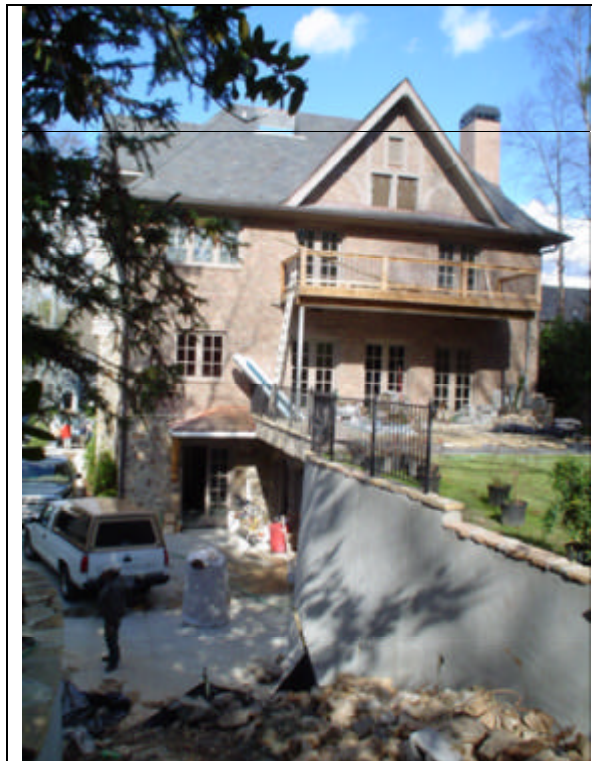
Installation of green area above 3-car garage.
