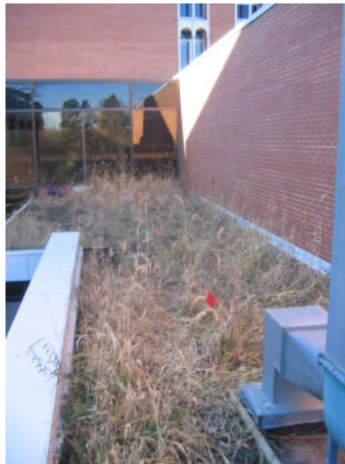
The green roof as viewed from Plot I (see Figure 1 below). The red flags pictured help mark the plot boundaries.
