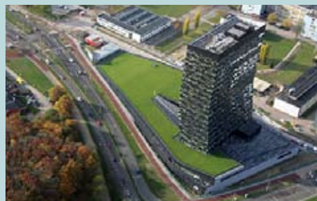
FiftyTwoDegrees (Nijmegen) – Natural stormwater management with green roofs
