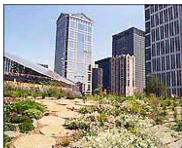
Shrubs and plants on top of Chicago's City Hall are expected to save the city up to $5,000 a year in heating and cooling bills. (City of Chicago)
